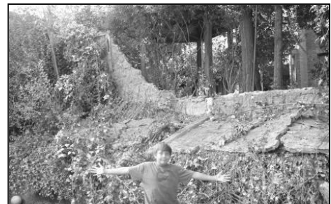
Vivian's son looks at the damage in his yard.
